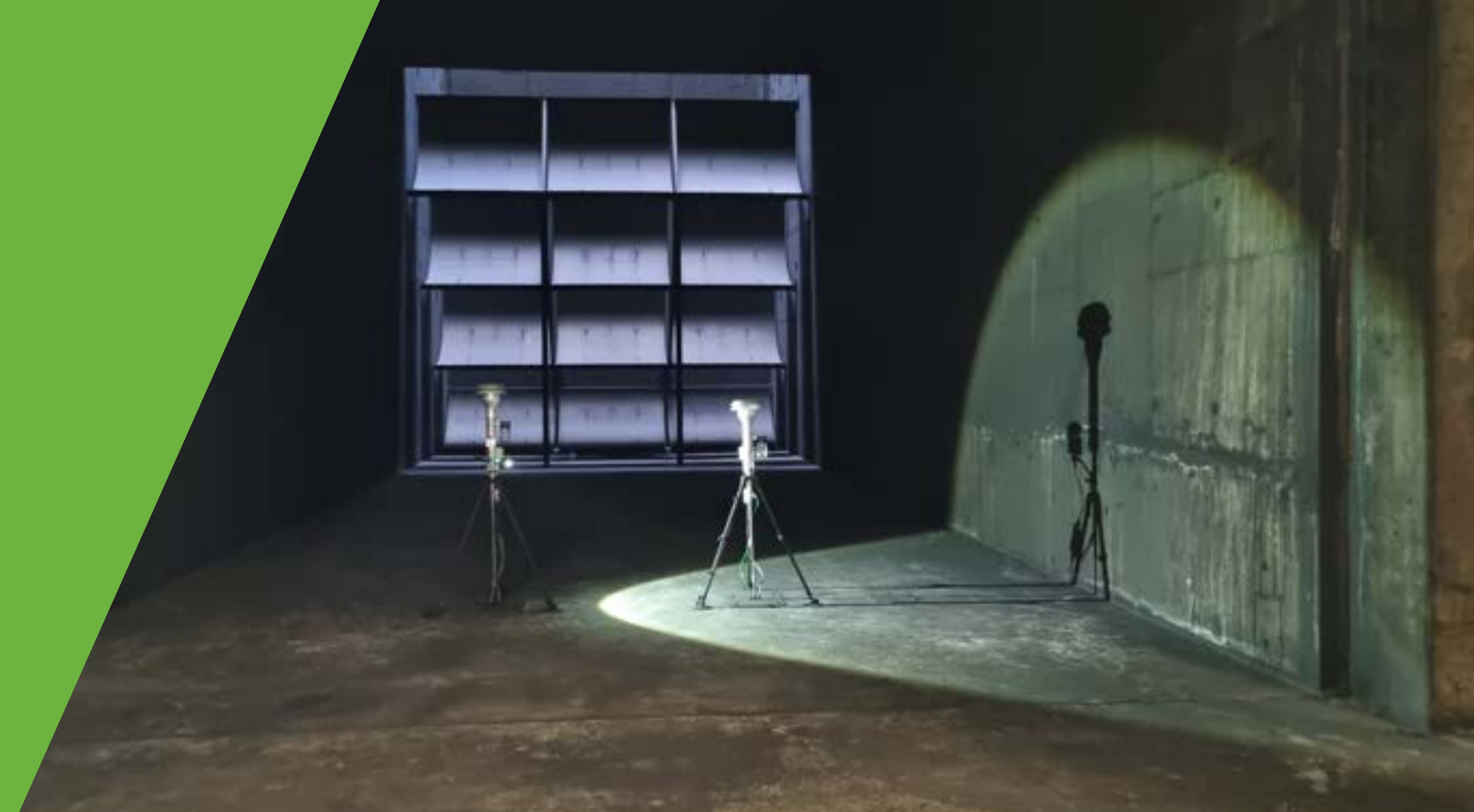
New particulate matter sensors (Above) located within the plenum of the Mullum Mullum ventilation stack, with the new control units located in the air quality monitoring cabinet (Below)
