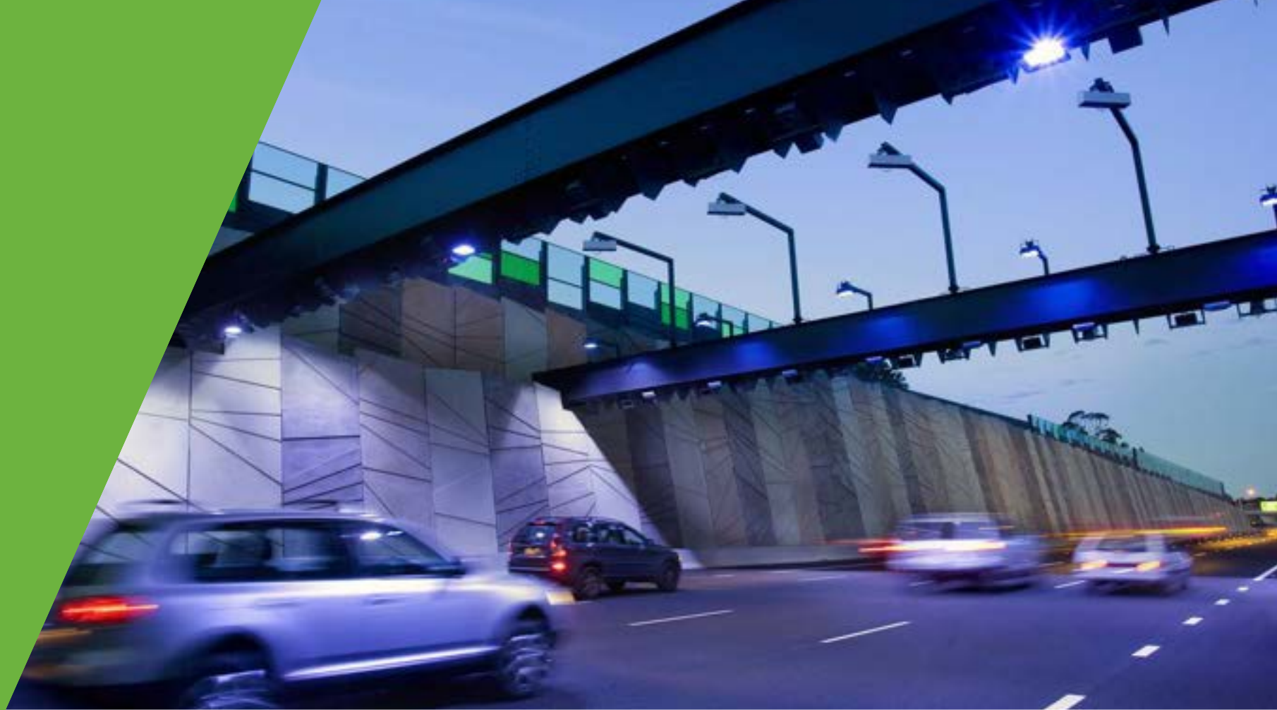
EastLink's imaging processing system uses digital images of passing vehicles to process tolls for customers without tags.
