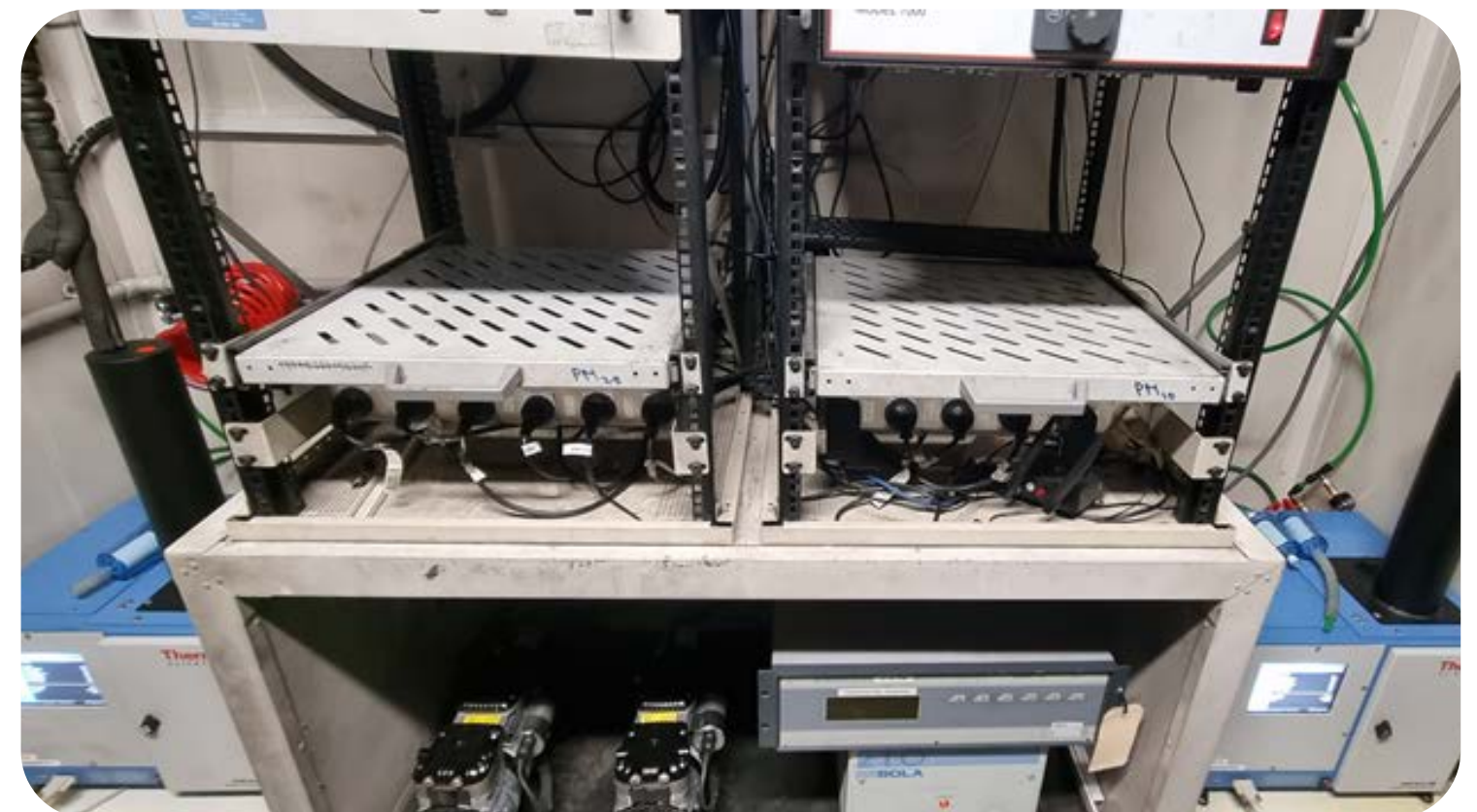
New particulate matter sensors (Above) located within the plenum of the Mullum Mullum ventilation stack, with the new control units located in the air quality monitoring cabinet (Below)
